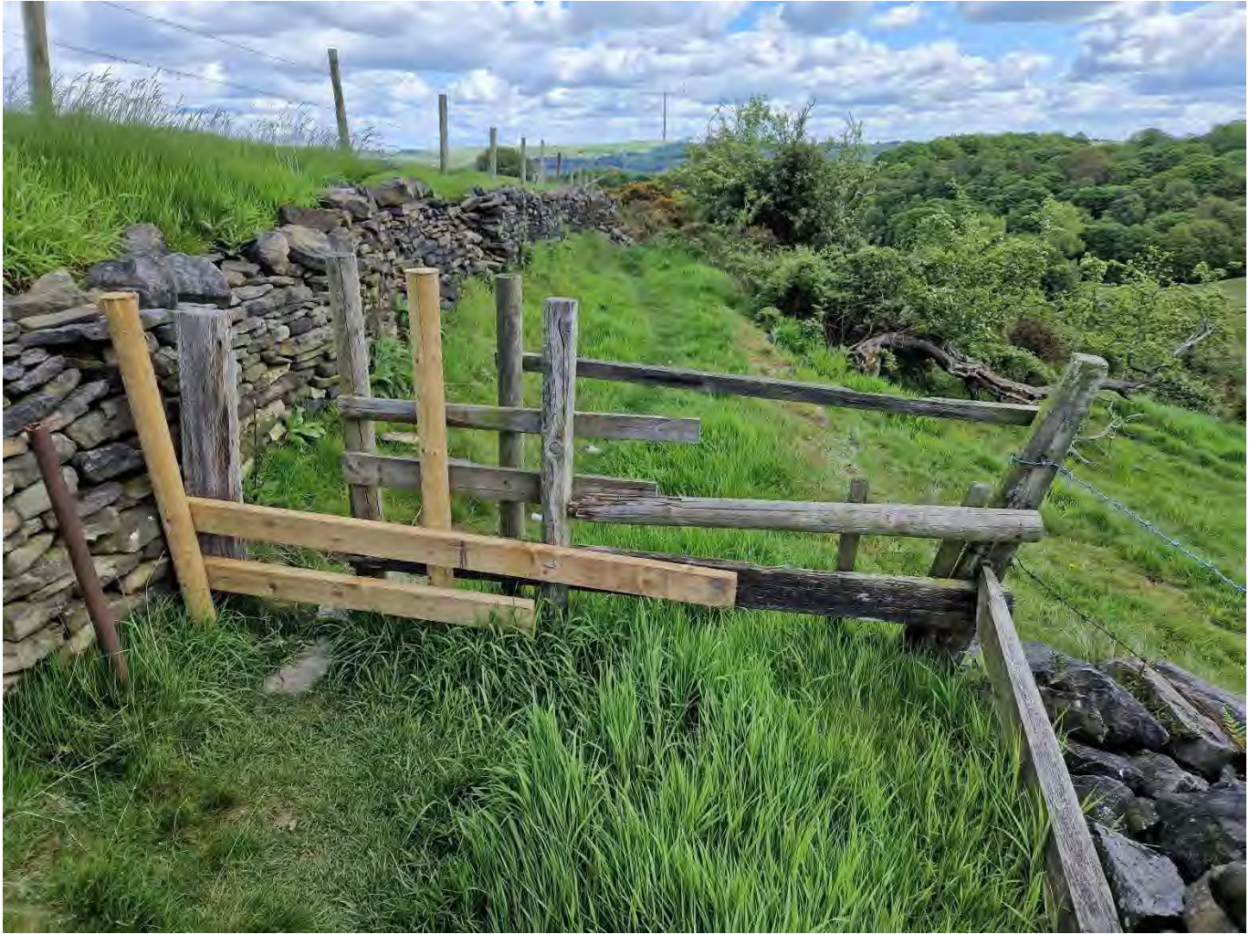
Photo 13: Close-up of second wooden stile structure.
